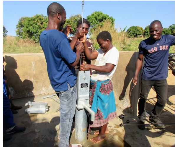
Members of the water point committee are taught how to maintain the new installation
